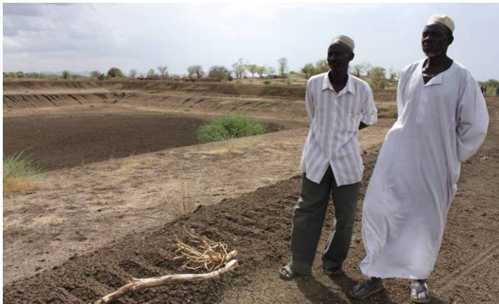
SOS Sahel rehabilitated this large (30,000 cubic metre capacity) government-built hafir at Kolandy Village, South Kordofan. © Lucy Polson/SOS Sahel UK
